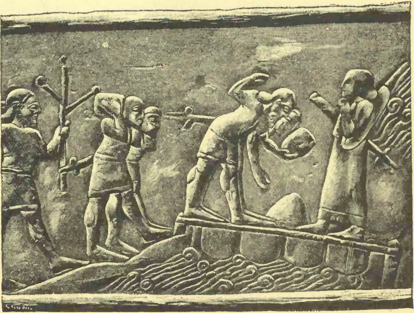
MAKING A BRIDGE FOR THE PASSAGE OF THE CHARIOTS. 2
